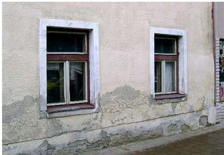
Fig. 1: Surface layer destroyed by moisture
